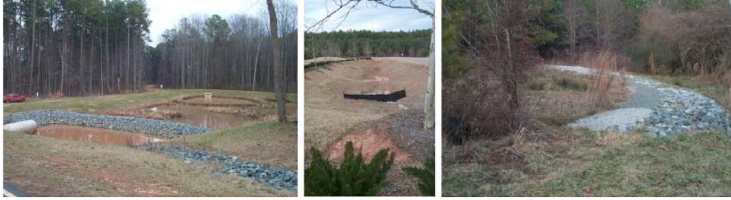
Figure 7: Sediment control measures (wetland, fence, check dam)
